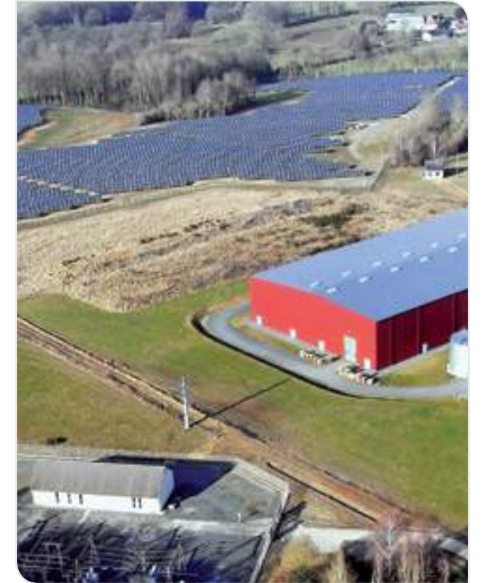
Bonnat, France PV power plant 5.4 MW
