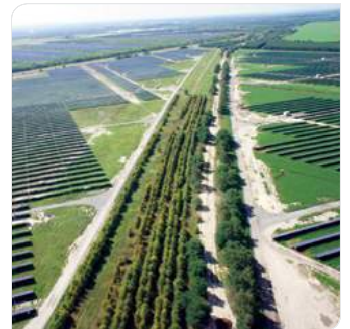
Senftenberg, Germany PV power plant 82 MW
