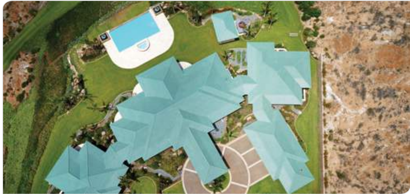
Maui, USA Off-grid solar (ground mounted PV arrays) 20 kW
