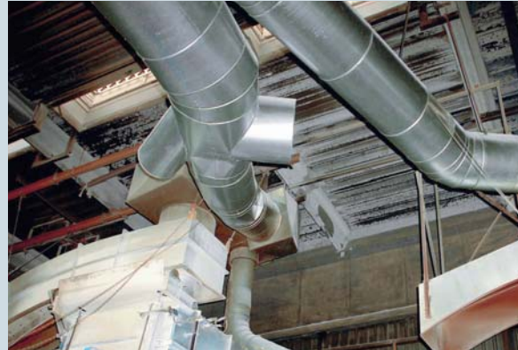
Frequency converters permit 66 % energy savings in a flue-gas filter system at Siemens
