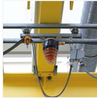
Cranes & loading equipment
